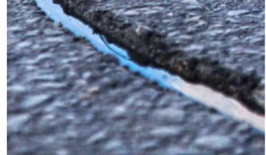
IS-COAT is an insulant material that is applied hot, and it does not produce air bubbles and ruptures when heated up; and through its consistent flow, it maintains consistency to be poured in a way that completely fills up the area of application. It prevents influx of water from cracks in between the asphalt coatings, and this way removes problems caused by water and humidity.
