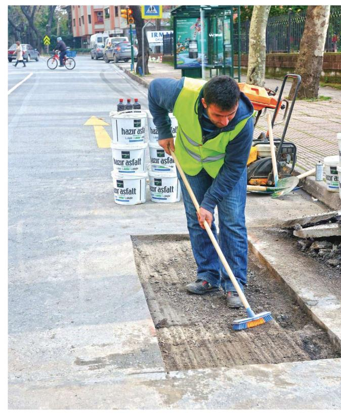
Ready Asphalt is a cold asphalt mix that can be processed even in cold weathers, and it is used to repair potholes. It is the kind of mixed cold asphalt that is practically used in repairing the potholes and deteriorations on concrete and asphalt surfaces, with no need for heat or compression. It is used in urban roads, express ways, factories, hospitals, schools, hotels, recreational facilities, playgrounds, indoor and outdoor parking lots, as well as in
